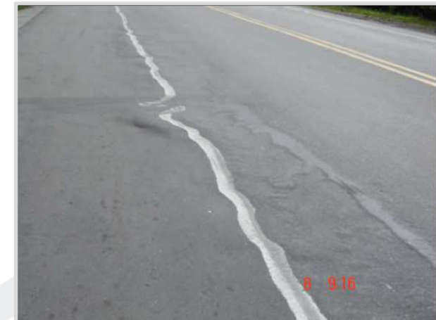
Pavement deformation (asphalt exudate) Source: http://hechosdetransito.com
