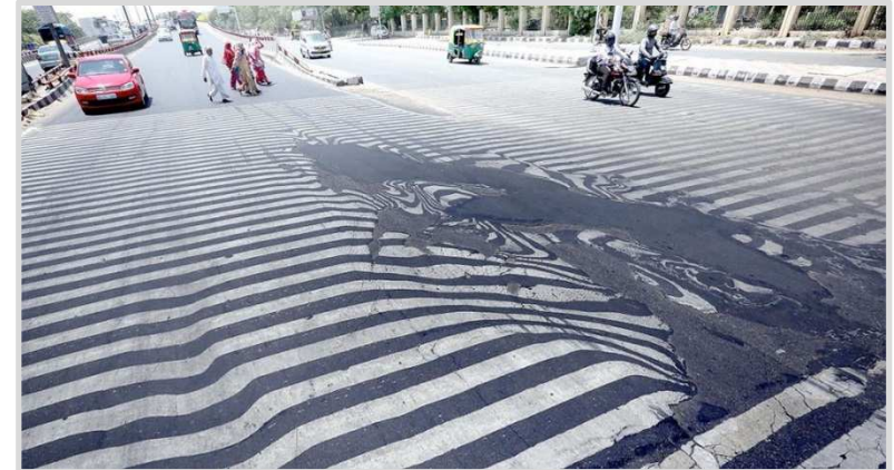
Deformation of urban pavement in India Source: http://i.ngenespanol.com/
